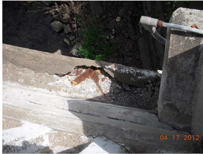
SPALL WITH EXPOSED LATTICE STEEL ON TOP OF ARCH SOUTH SIDE AT WEST ABUTMENT
