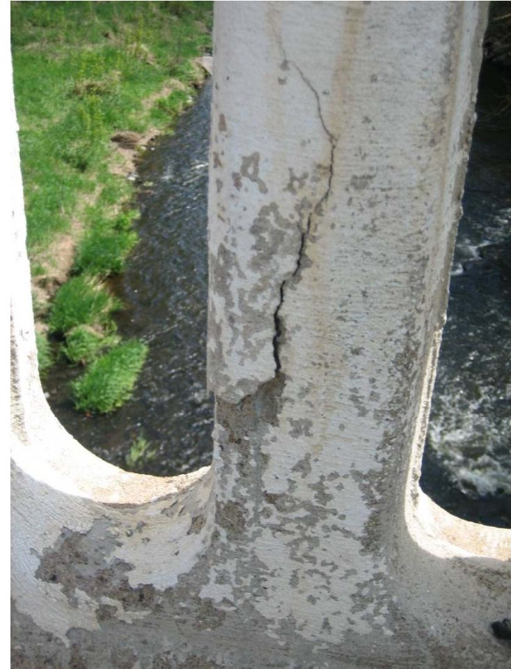
SPALL & CRACK ON FRONT FACE OF RAILING VERTICAL ON SOUTH SIDE OF BRIDGE
