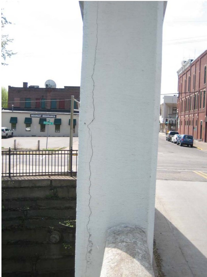
CRACK ON INSIDE FACE OF HANGER ON SOUTH SIDE OF BRIDGE
