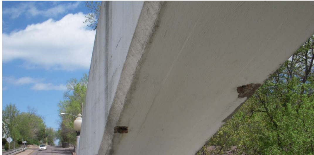
SPALLS WITH EXPOSED REBAR ON BOTTOM OF ARCH ON SOUTH SIDE OF BRIDGE
