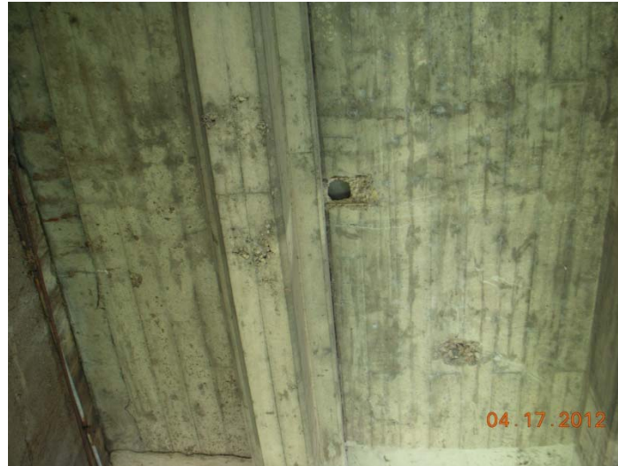
HOLE AND SPALL ON BOTTOM OF DECK
