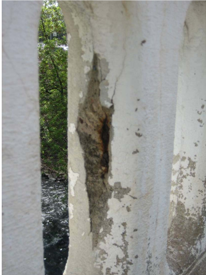
SPALL ON INSIDE FACE OF RAILING VERTICAL ON SOUTH SIDE OF BRIDGE
