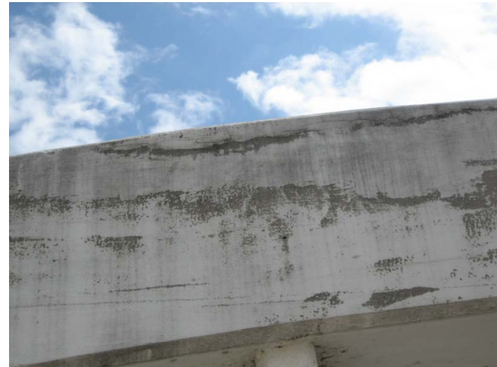
CRACKS ON FRONT OF ARCH TOP AND BOTTOM ON SOUTH SIDE OF BRIDGE
