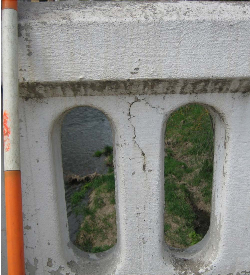
CRACK ON FRONT OF RAILING VERTICAL ON NORTH SIDE OF BRIDGE
