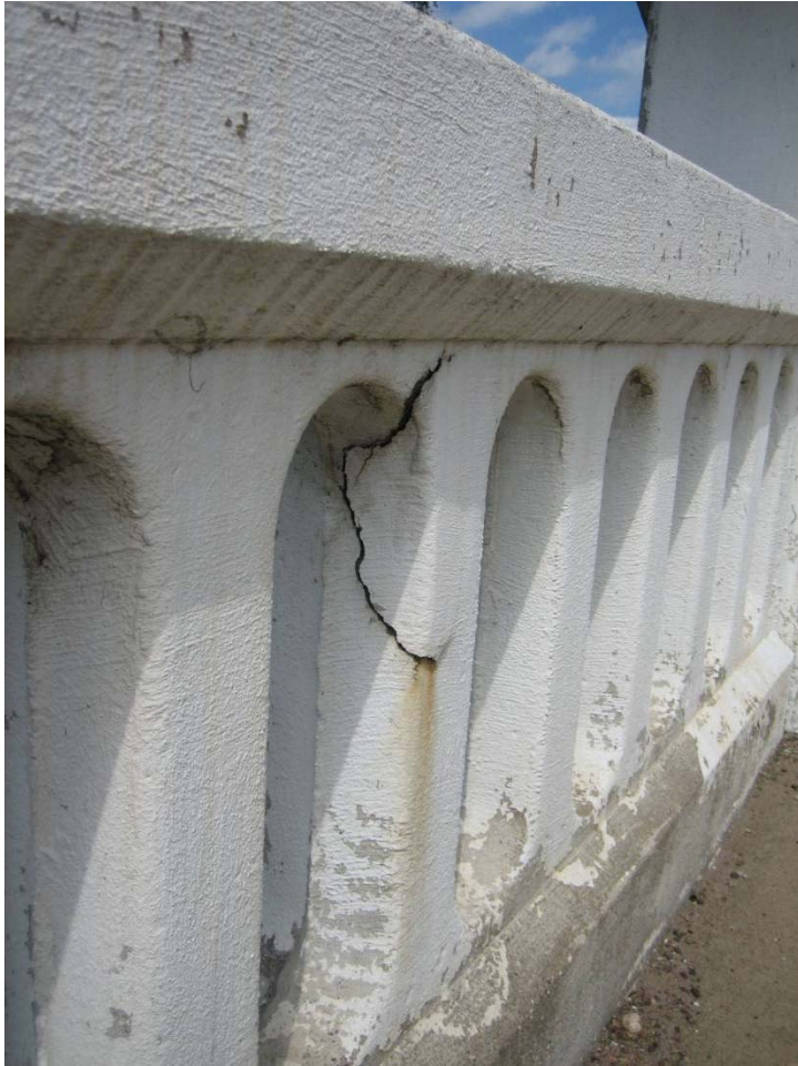
CRACK ON INSIDE FACE OF RAILING VERTICAL ON NORTH SIDE OF BRIDGE
