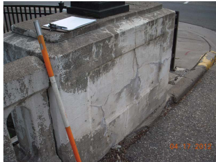
CRACKS ON FRONT OF END BLOCK CONCRETE RAILING ON SOUTH SIDE OF BRIDGE
