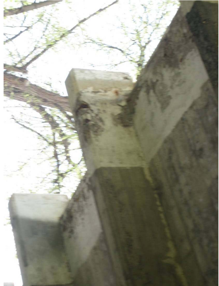
DISTRESSED CONCRETE END OF FLOOR BEAM ON SOUTH SIDE OF BRIDGE
