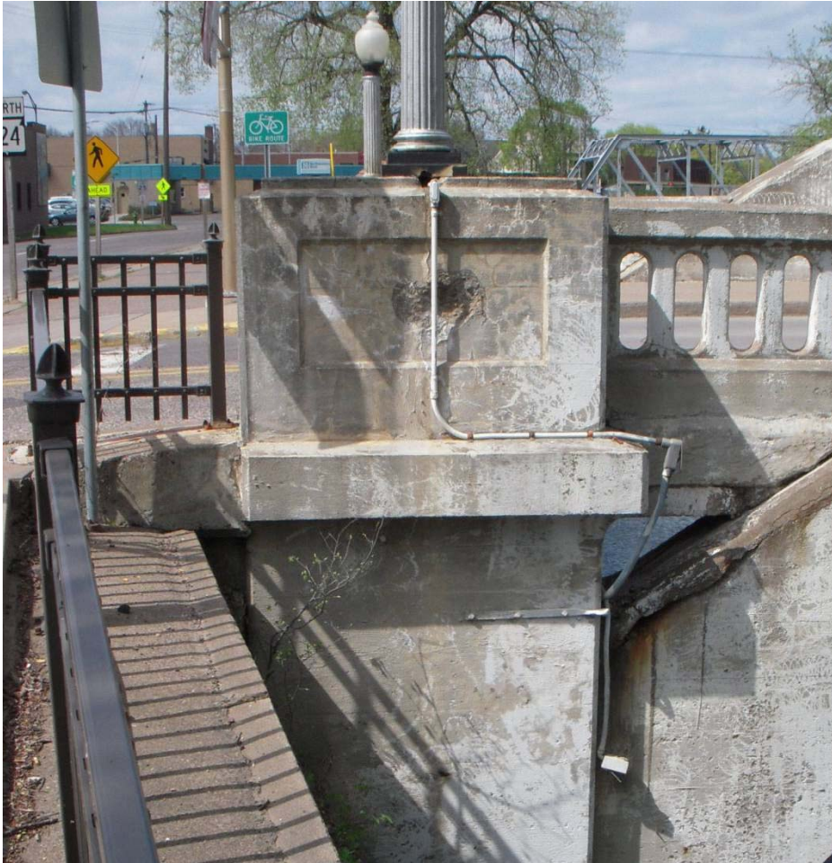
SPALL ON BACK OF END BLOCK CONCRETE RAILING ON SOUTH SIDE OF BRIDGE
