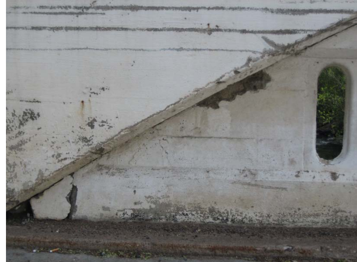
SPALLED CONCRETE ON FRONT OF RAILING ON SOUTH SIDE OF BRIDGE
