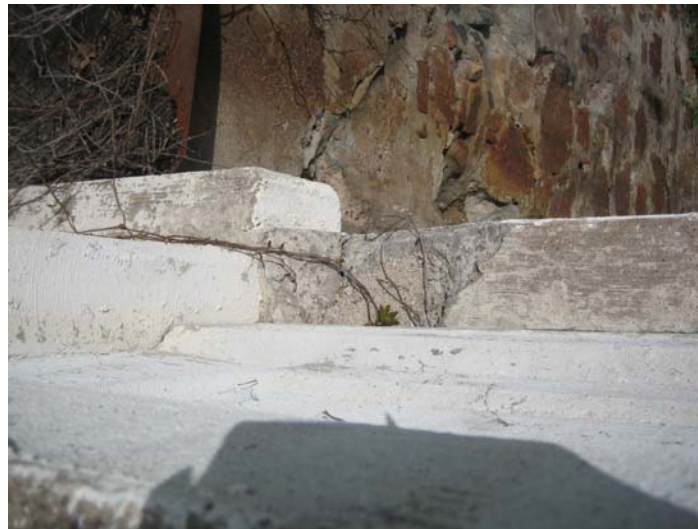
SPALL ON TOP OF ARCH SOUTHSIDE AT EAST ABUTMENT
