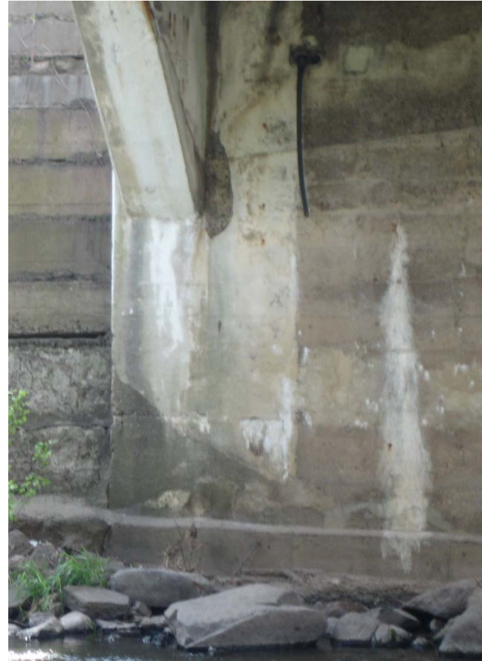
CRACK ON BOTTOM OF FRONT OF ARCH ON SOUTHSIDE OF BRIDGE WEST SIDE
