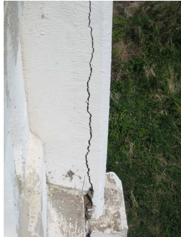
CRACK ON INSIDE FACE OF HANGER ON SOUTH SIDE OF BRIDGE
