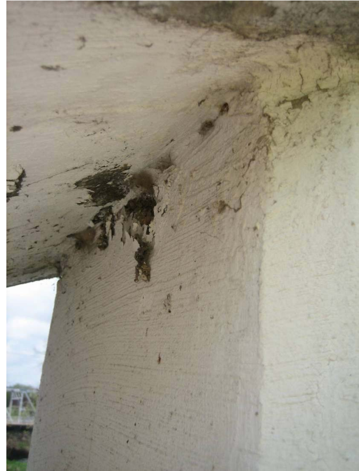
SPALL AT JOINT OF ARCH AND HANGER ON NORTH SIDE OF BRIDGE
