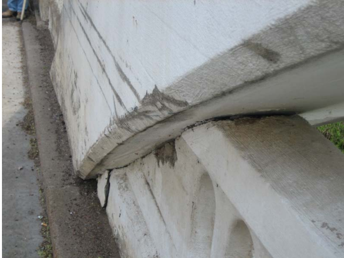
SPALLED CONCRETE ON FRONT OF RAILING ON SOUTH SIDE OF BRIDGE
