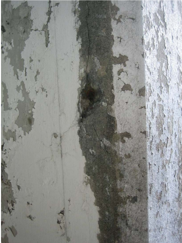
CRACK ON INSIDE FACE OF HANGER ON NORTH SIDE OF BRIDGE
