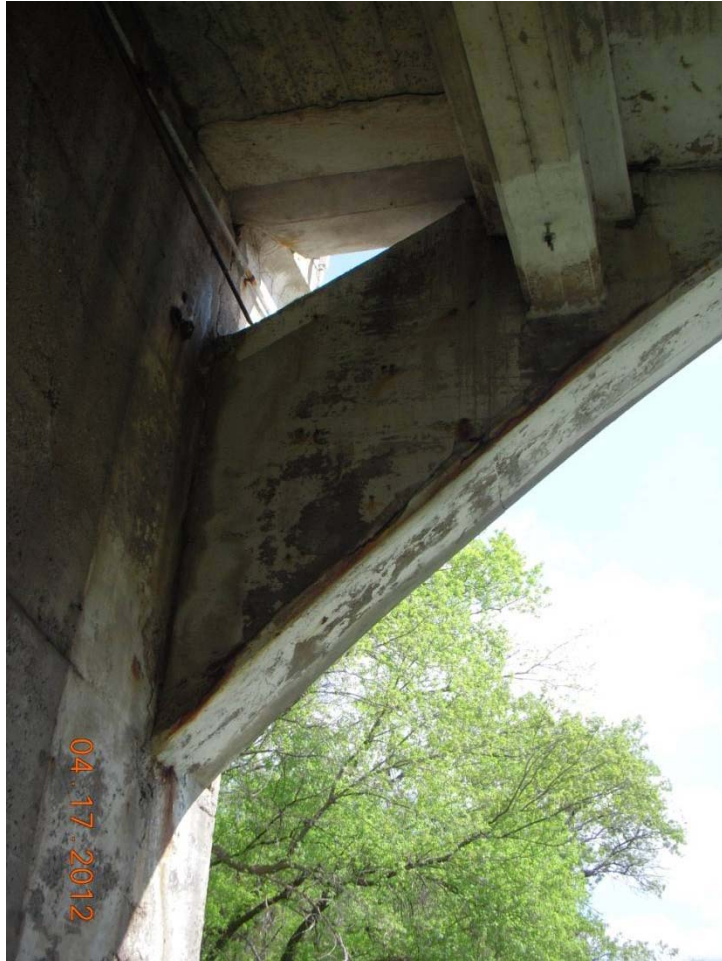
CRACK ON BOTTOM OF FRONT OF ARCH ON SOUTHSIDE OF BRIDGE EAST SIDE
