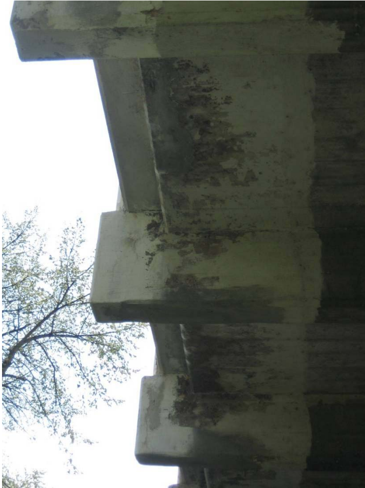
DISTRESSED CONCRETE END OF FLOOR BEAMS ON SOUTH SIDE OF BRIDGE
