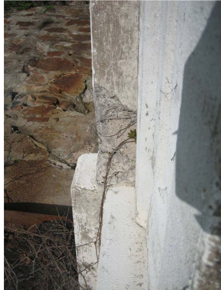
SPALL ON TOP OF ARCH ON SOUTH SIDE OF BRIDGE
