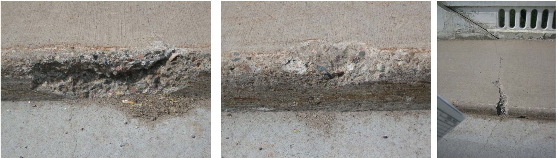
SPALLS AND CRACK ON INSIDE FACE OF SIDEWALK ON NORTHSIDE OF BRIDGE
