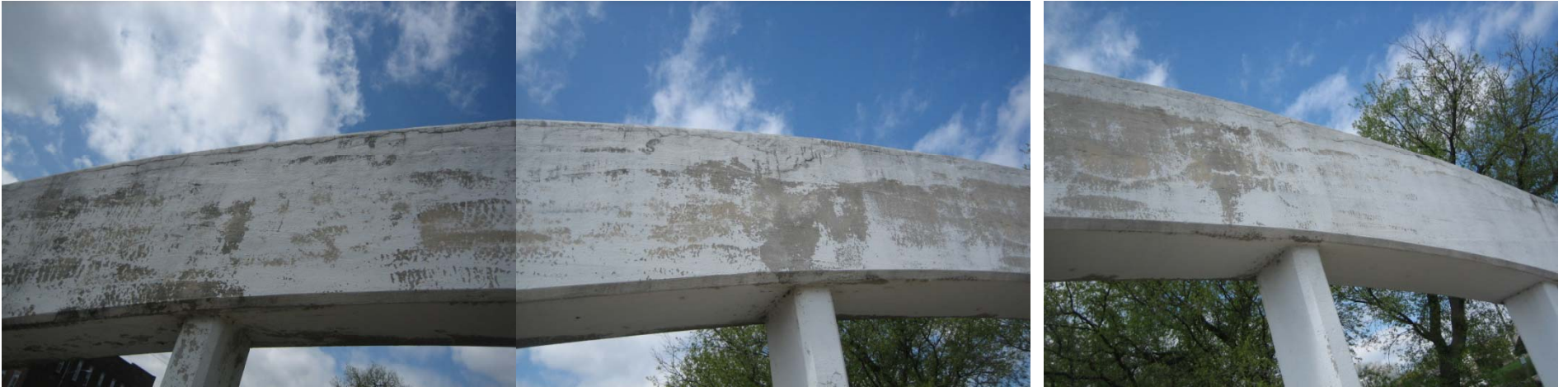
CRACK ON TOP OF FRONT OF ARCH ON NORTH SIDE OF BRIDGE
