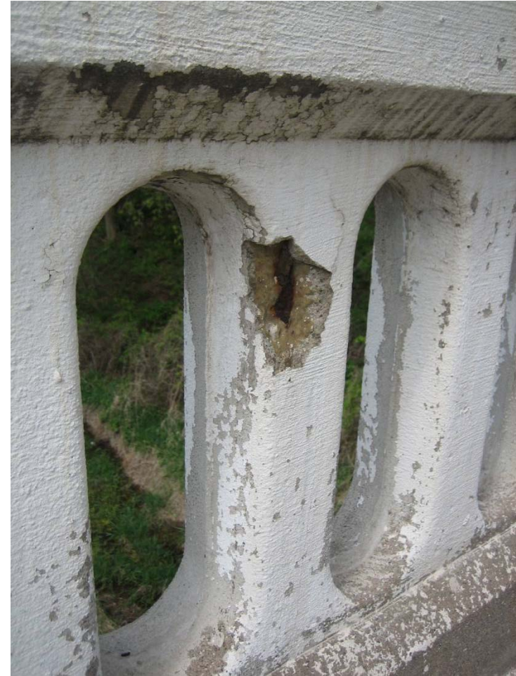
SPALL WITH EXPOSED REBAR ON FRONT OF RAILING VERTICAL ON NORTH SIDE OF BRIDGE
