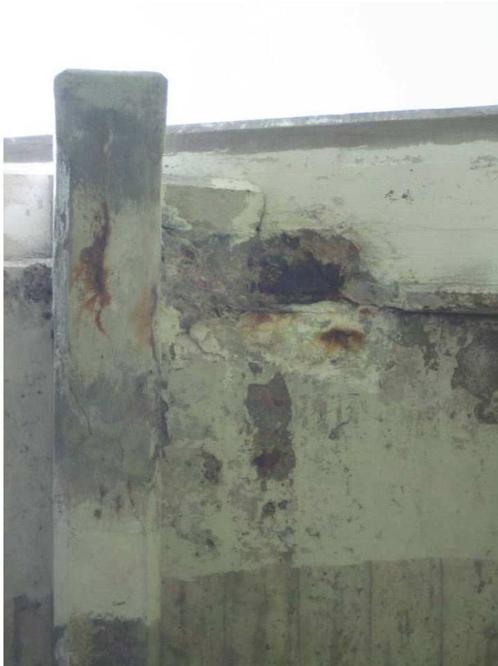
SPALL ON BOTTOM OF ARCH NEAR FLOOR BEAM ON SOUTH SIDE OF BRIDGE
