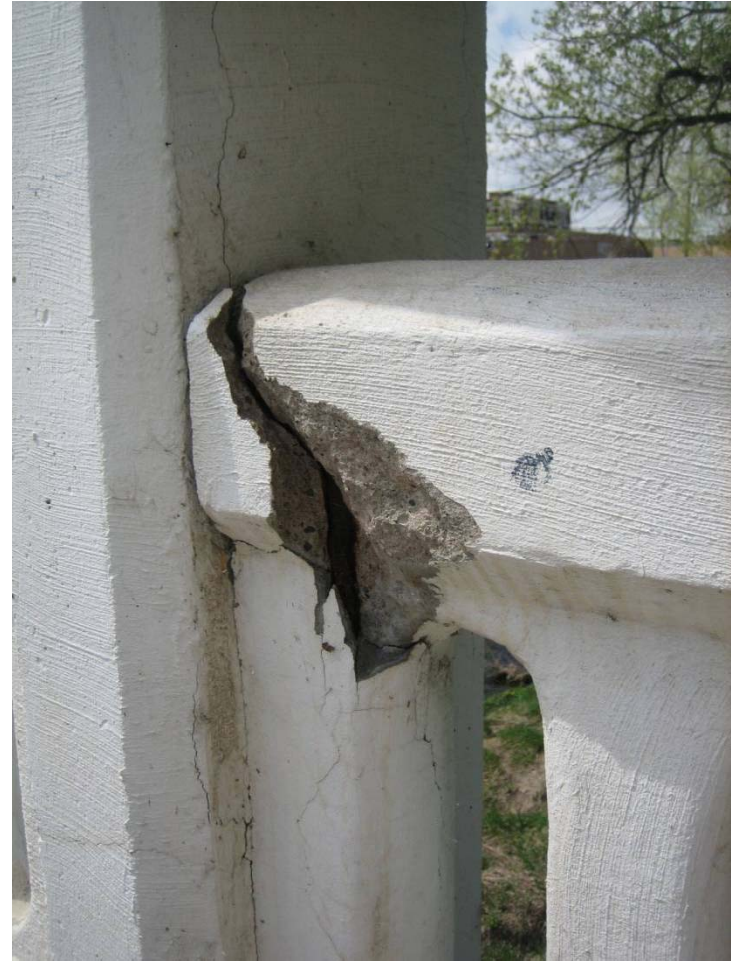
SPALL ON FRONT OF RAILING ON NORTH SIDE OF BRIDGE
