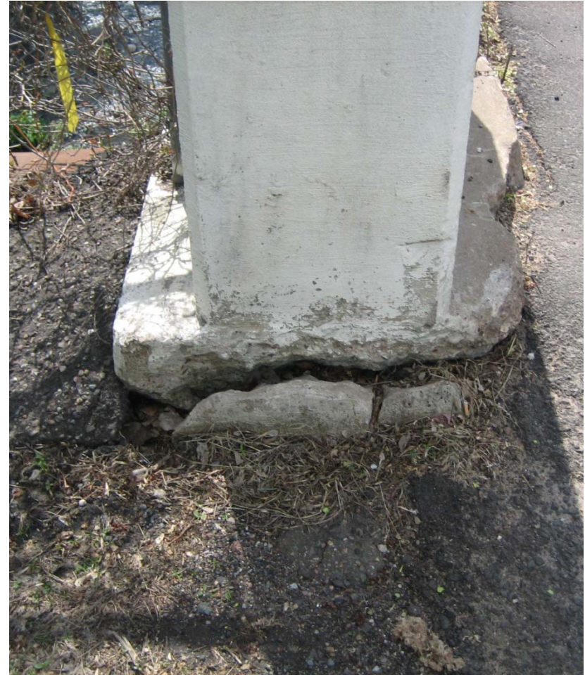
SPALLED CONCRETE ON BOTTOM OF ARCH ON SOUTH SIDE OF BRIDGE
