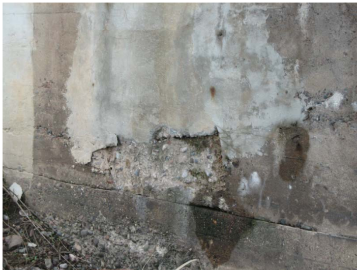
SPALLS AND CRACKS ON THE NORTH EAST ABUTMENT
