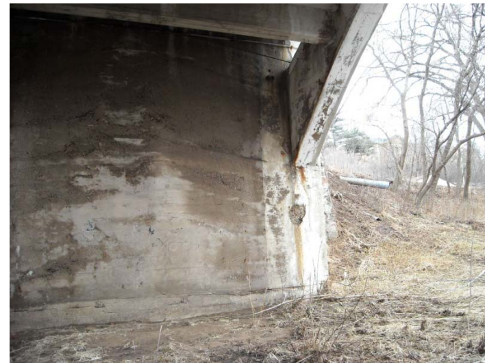
SPALLS AND CRACKS ON THE NORTH EAST ABUTMENT
