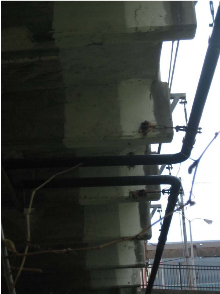
DISTRESSED CONCRETE END OF FLOOR BEAMS ON NORTH SIDE OF BRIDGE
